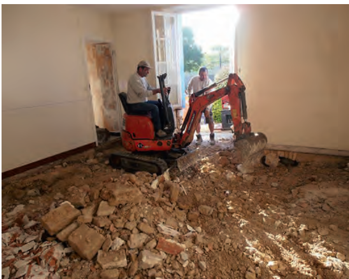
PREPARATION SOL SECRETARIAT
